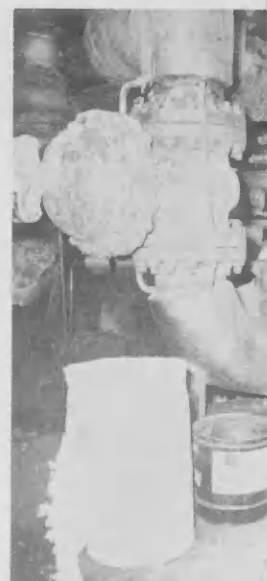
Antonio Schwengle (rear) of the "hottest" fittings wool blanket
